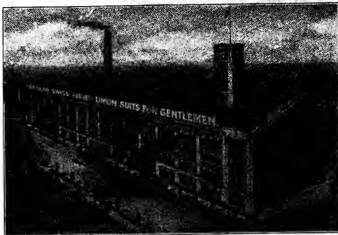
NEW PLANT OF VASSAR SWISS UNDERWEAR CO., CHICAGO, ILL.
